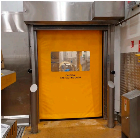
Up to 2.0m/sec. with the standard frequency control
